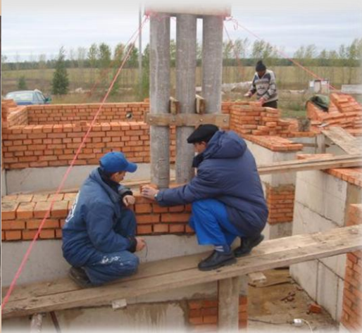
Masonry Chimney Construction
